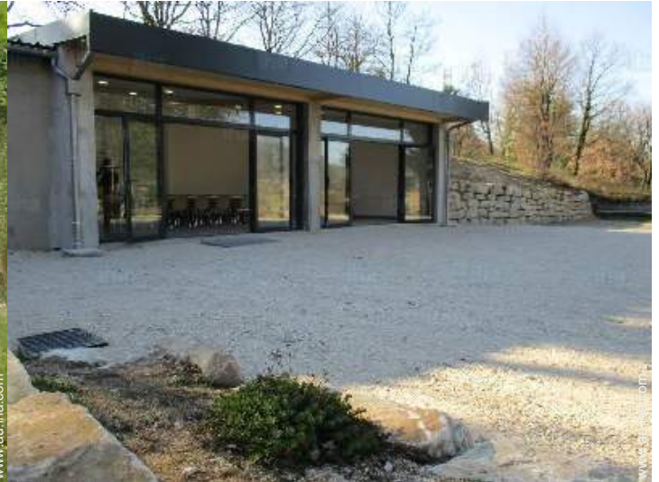
Equipment at the guest's disposal
